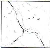
Cracks in stone
